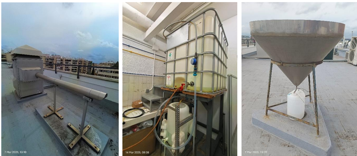
Environmental radioactivity monitoring facilities, including high-flow air samplers with 4 ft × 4 ft filters, large-volume water tanks for routine surveillance of gamma-emitting radionuclides in drinking water, and rainwater samplers.
